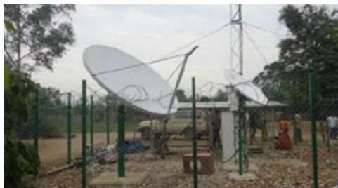
Secure installation of solar-powered, satellite-enabled, mobile base station
