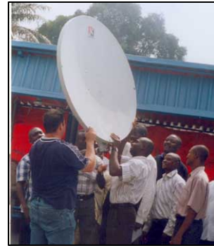
Installing VSAT equipment
